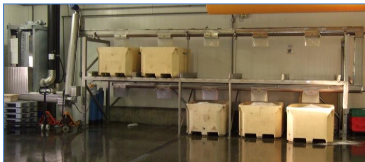
Ice storage. Flake ice from the V316 iceflaker is transported to insulated bins by ançers.
